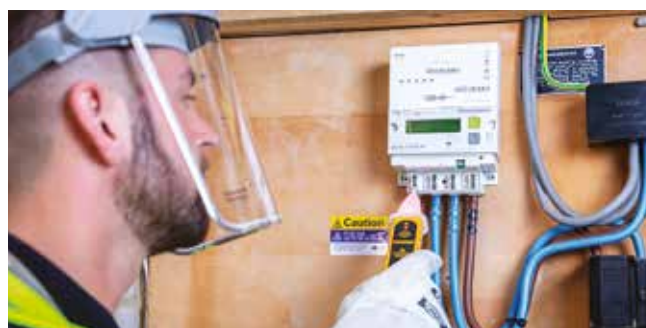
Safety first: Vital PPE kit protects engineers
